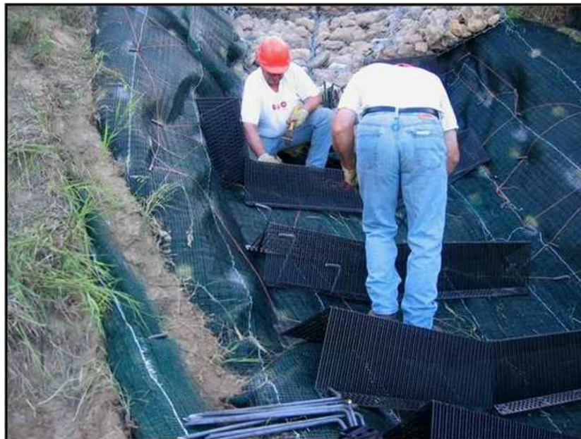
BMP # 6 EROSION CONTROL BLANKET - DITCH * (2 OF 2)
