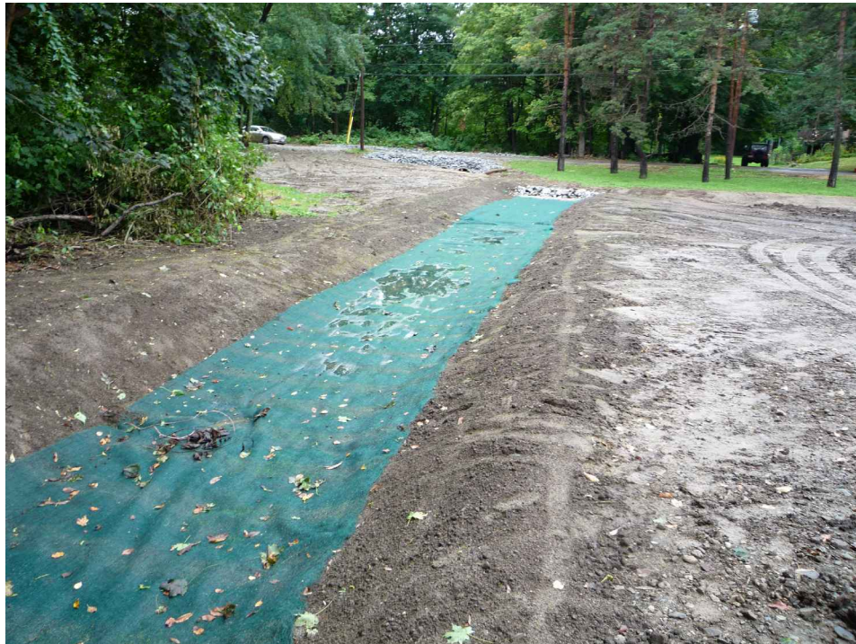
BMP # 29 DRAINAGE SWALE AND LINED DITCH
